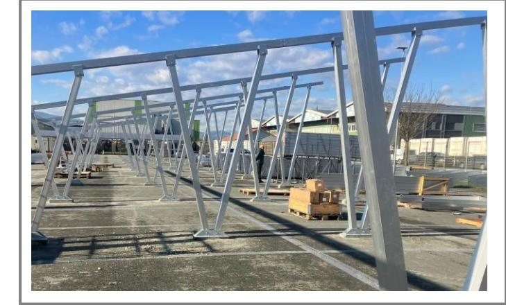
Solar PV car park canopies generate significant solar power (c.5-6kWp per 2 bays) for use at site and/or perhaps as EV charging in conjunction with a battery storage system.
