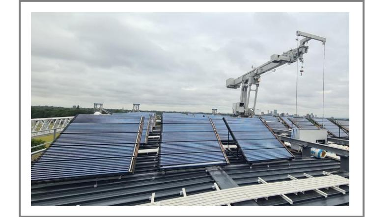
LaZer2 solar thermal is specifically designed to produce hot water.
