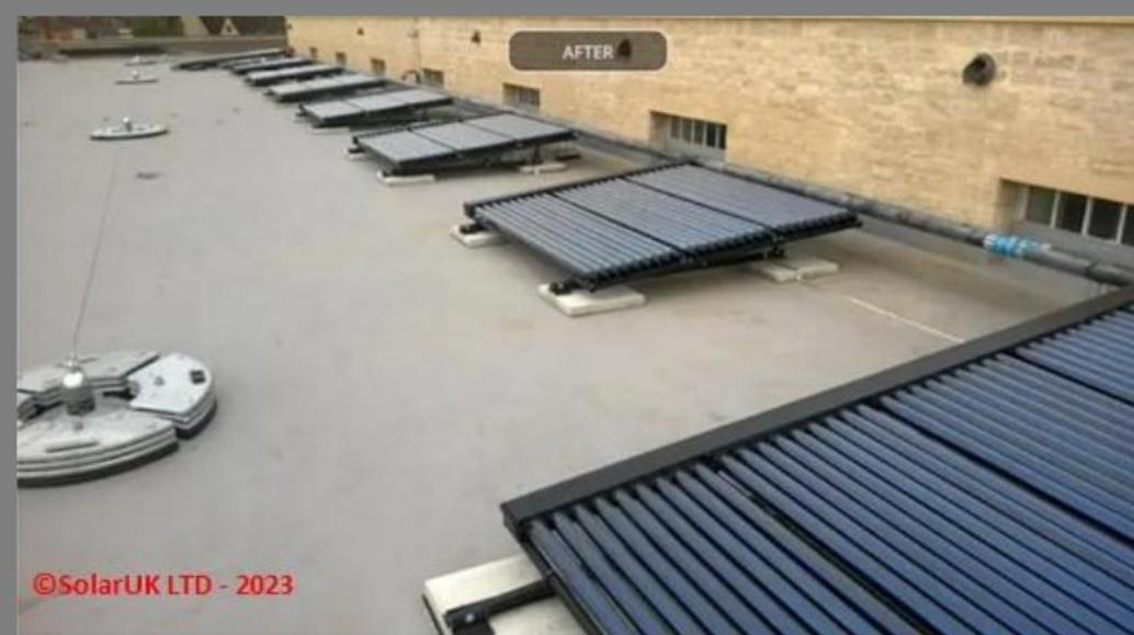
We designed, supplied, and installed 25m<sup>2</sup> of LaZer2 solar thermal collectors, feeding into the site's DHW infrastructure, providing 21MWh·th of hot water and reducing the reliance on gas. Our 3-man team led by lead LaZer2 installation engineer, Nick Martyn, and project managed by our Technical Director, Duncan Lee, installed and commissioned the system in c.6 weeks.
