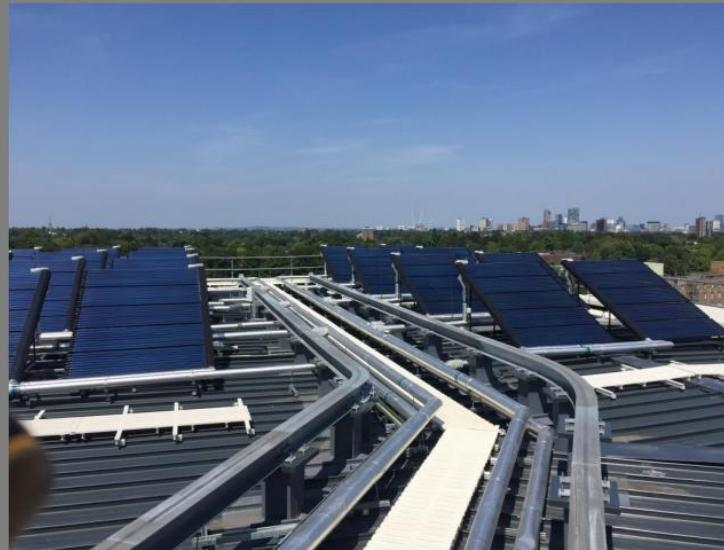
For this site, we supplied and installed 100m<sup>2</sup> of LaZer2 solar thermal collectors, feeding into the site's LTHW infrastructure, providing 50.9MWh-th of hot water and reducing the reliance on gas.
