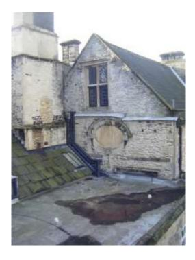
Solar pipework emerging from a flat roof was designed to be indistinguishable from the exiting black cast iron pipes.
